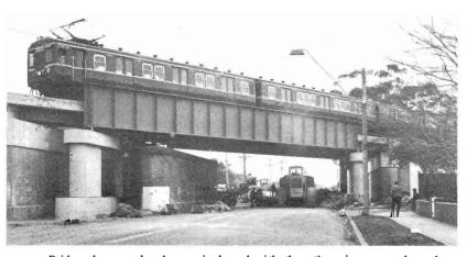
Bridge clearance has been raised, and with the other pier removed, road width will have been increased, too.
