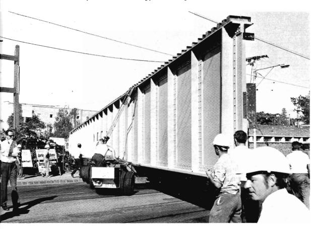
BIG SHIFT. For the final stage of the third track works between Burnley and Hawthorn (October 1971 News Letter, p. 150), two 150 ft. long, 70 ton girders were delivered on March 19 to Hawthorn station. Too large for some rail curves in the area, they were taken to Hawthorn by road where the delicate manoeuvres to get them into the rail yard held the attention of all.
