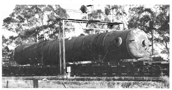
BIG HAUL FOR BIG LOAD. More than 1,300 miles of rail travel was in store for this huge absorber vessel bound for the Gidgealpa oil and gas field in outback South Australia. The 140-ton vessel was travelling from Melbourne to Telford, S.A., via Albury, Parkes, Broken Hill, Peterborough and Port Augusta to avoid transfers – this route is standard gauge all the way. The vessel was photographed at Violet Town on September 4.
