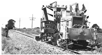
to lift, pack and line the track. Annually, about \$16 million is spent on this type of work which maintains and upgrades the State's railway network. Incidentally, that puff of smoke under the front wheels of the locomotive was caused by a detonator on the track to warn other workmen in the area.
