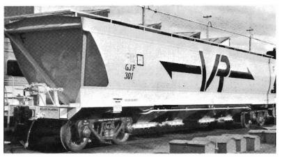
A job well done. The finished article ready for traffic, one of 350 bogie hopper wagons of which Newport built 150.
