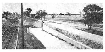
Whenever possible, and appropriate, the new standard gauge line was grade-separated. At Springhurst a flyover takes the line over the station access road.
