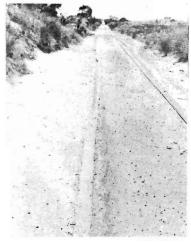
Despite a train the previous day and heavy overnight rain, the Mallee sand can quickly claim the railway area.
