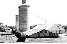
More than 800,000 bushels of grain can be stored in Rainbow's silos. The rear concrete silo is air-conditioned.
