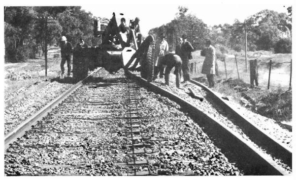
RELAYING of the 281-mile Ballarat-Mildura line is now in its final stages, with work concentrated in the Maryborough area. Assisting with the heavy work of placing 225-ft. lengths of welded 94-lb. rail is a machine recently purchased from Silverton Rail Services after upgrading work on the Kalgoorlie-Esperance line in Western Australia. The machine, called a *Speedswing*, rapidly positions the three-ton rails ready for spiking by following mechanised gangs.
