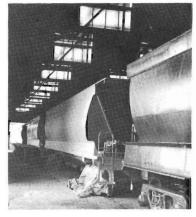
In the paint shop, wagons go through the following stages over the three days (from right): de-oxidine, primer, undercoat, finishing coat.
