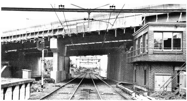
ROOF ROAD. Road widening works at the West Footscray overpass of Geelong Road, (known to locals as Mount Mistake) encroached on the railway signal box area. Rather than move the box, the tiled, gable roof was whipped off, and a flat roof provided.
