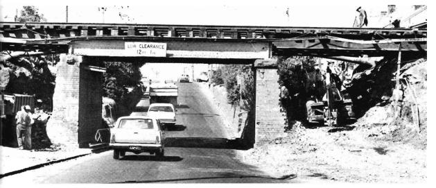
WIDER. A well-known traffic bottleneck, the narrow bridge under the railway at Francis Street, Yarraville, is being widened by V.R.'s Special Works section at Council and C.R.B. expense. When finished, the road will be 50 ft. wide instead of 20 ft. The existing brick bridge abutments will be removed and new ones built at the footpath line, a pedestrian "tunnel" being provided through the abutments.
