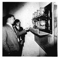
Chief Electrical Engineer, Mr. Alan Firth, explains the working of the drainage equipment inside a substation to News Letter Editor. The equipment feeds the current back into the circuit.
