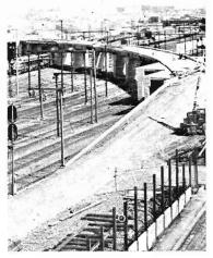
Because the standard gauge line uses the former metropolitan goods lines into Dynon for its approach to Melbourne, a new route into the city terminal, crossing the entire Melbourne Yard arrival area and western suburban lines, had to be found. A 13-pier curving concrete flyover brings the line into correct position for the run into Nos. 1 and 2 Platforms at Spencer Street.
