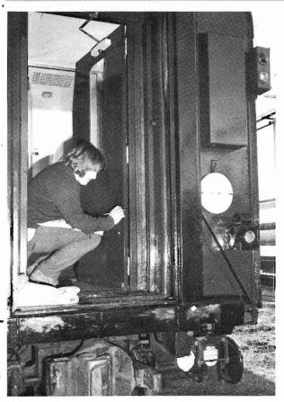
MODIFIED. For *The Vinelander* two twinettes and two roomettes from *The Overland* have been painted blue instead of maroon and modified for operation on the Mildura line. Seen renovating the draught seals on the vestibule door is Upholsterer Ian Burns.
