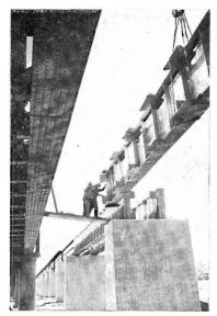
New bridges were built for the standard gauge line Wodonga and Broadmeadows. Clearly showing the changes in designs from the 1873-built broad gauge (left), is the new bridge for the 4 ft. 8½ in.
