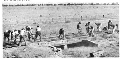
It's dry and dusty in the drought affected areas, and relaying a railway is heavy work. Presently, the 44 miles between Echuca and Deniliquin is being resleepered and sledded in prepararation for the relaying gangs. The Echuca Points and Crossing Gang plus the Utility Gang, and swelled by workers on drought relief, are seen here preparing the track for sledding just south of Moira station. The effect of the drought is obvious—this photo was taken at the end of October.
